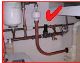
Compliant installation using hotun
